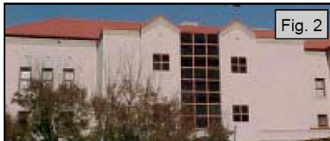
Fig. 1 shows utilities located on a roof and properly screened by parapet walls. Fig. 2 shows the effectiveness of that screening from the ground.
