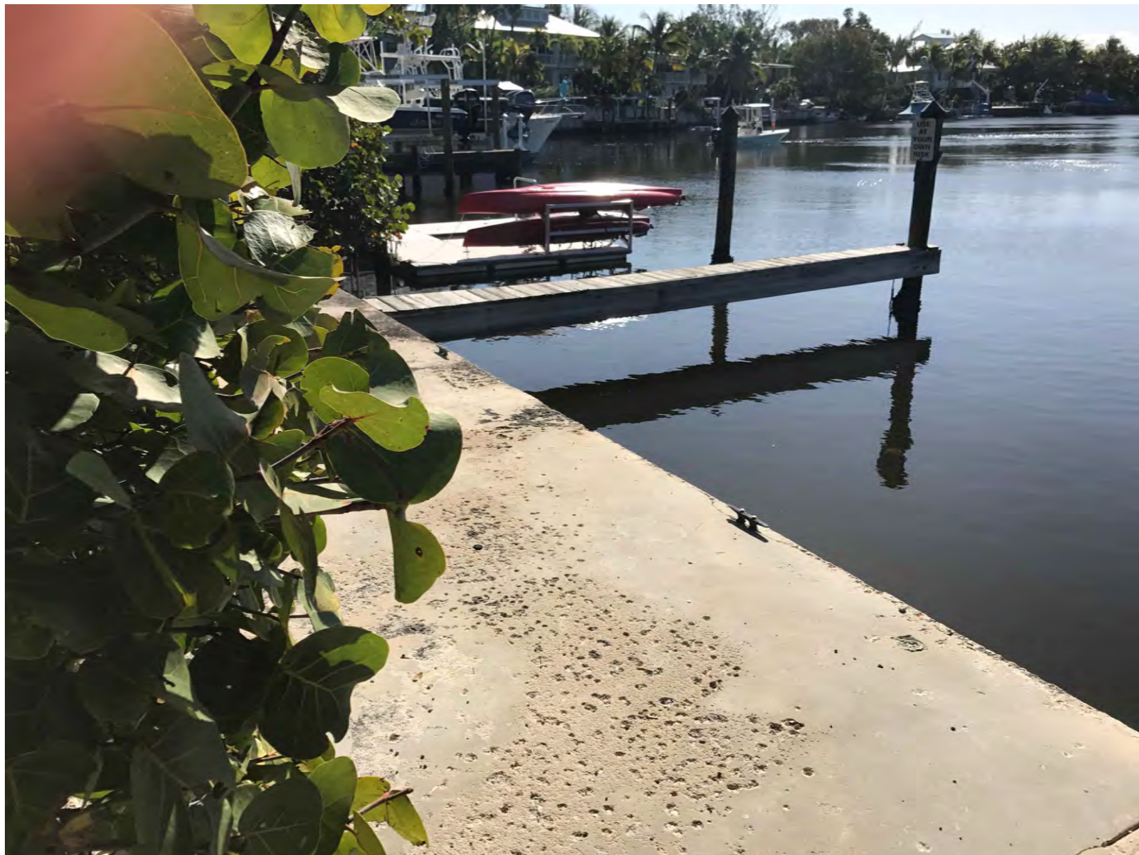
LIMESTONE SEAWALL WITH CONCRETE CAP AND ELEVATED WOODEN DOCK
