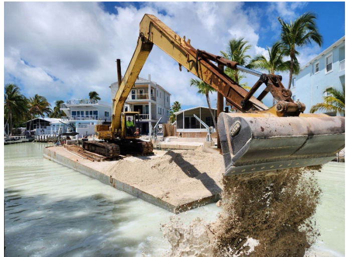
Photo: Canal 90 Backfill Operations
