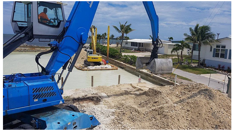
Photo: Canal 25 Backfilling
