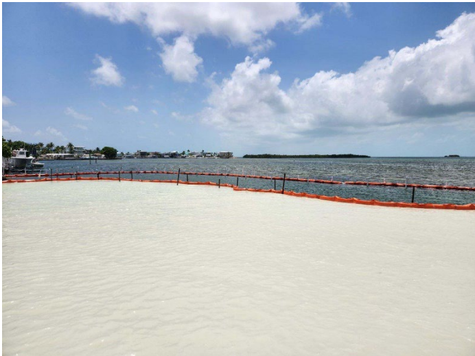
Photo: Canal 90 Turbidity Controls
