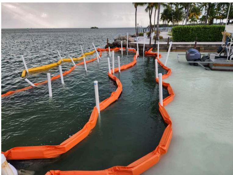
Photo: Canal 116 Turbidity Controls
