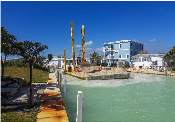
Photo: Canal 28 Backfilling
