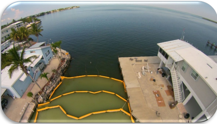
Photo: Canal 83 Turbidity Controls
