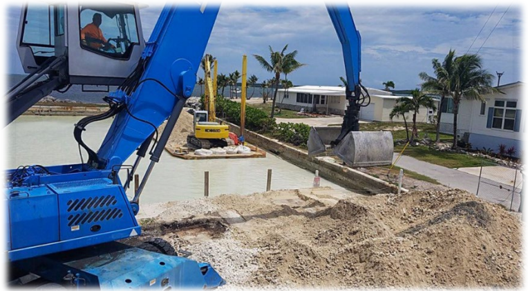
Photo: Canal 83 Organic Removal/Backfill Operations
