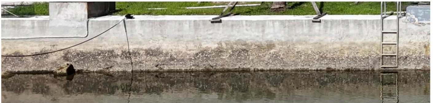
6417 Pine Tree Dr Circle: Precast Seawall - installed 1993
